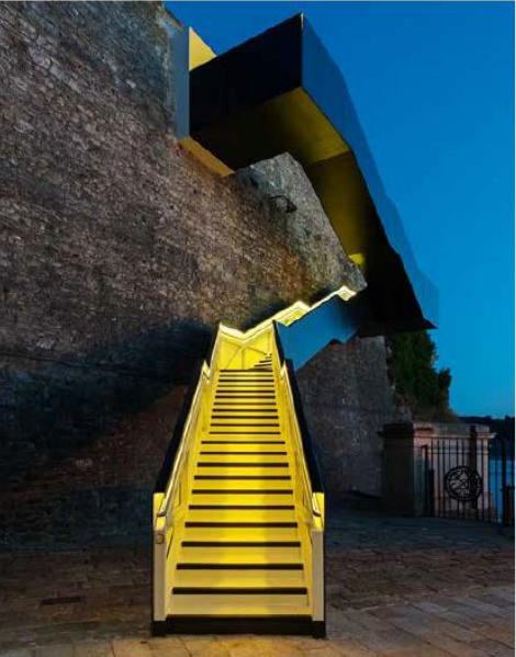
Figure 2.09: (And Below) Cantilevered stairs linking Royal William Yard in Plymouth to the public park above (Gillespie Yunnis Architects)
