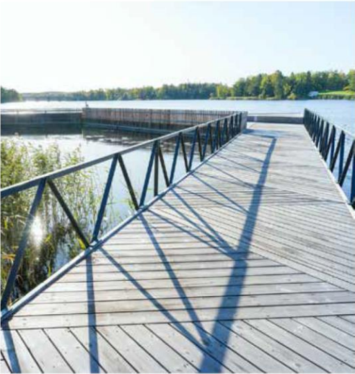
Figure 2.05: A new timber boardwalk opens up a recreational access to the lakeside of Lake Magelungen, Sweden. The boardwalk is a combination of a fixed structure attached to the land, connected by gangways to a floating pontoon construction. (Karavan landskapsarkitekt).
